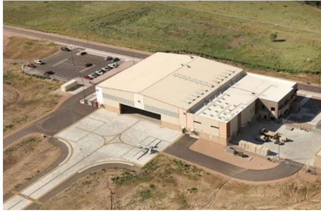
Unmanned Aerial Vehicle Hanger, Fort Carson
