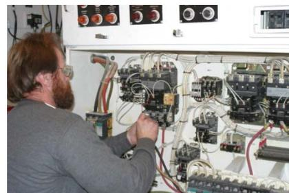
Sierra Army Depot mechanic performs repairs on the circuit breakers of a Reverse Osmosis Water Purification Unit during Reset.
